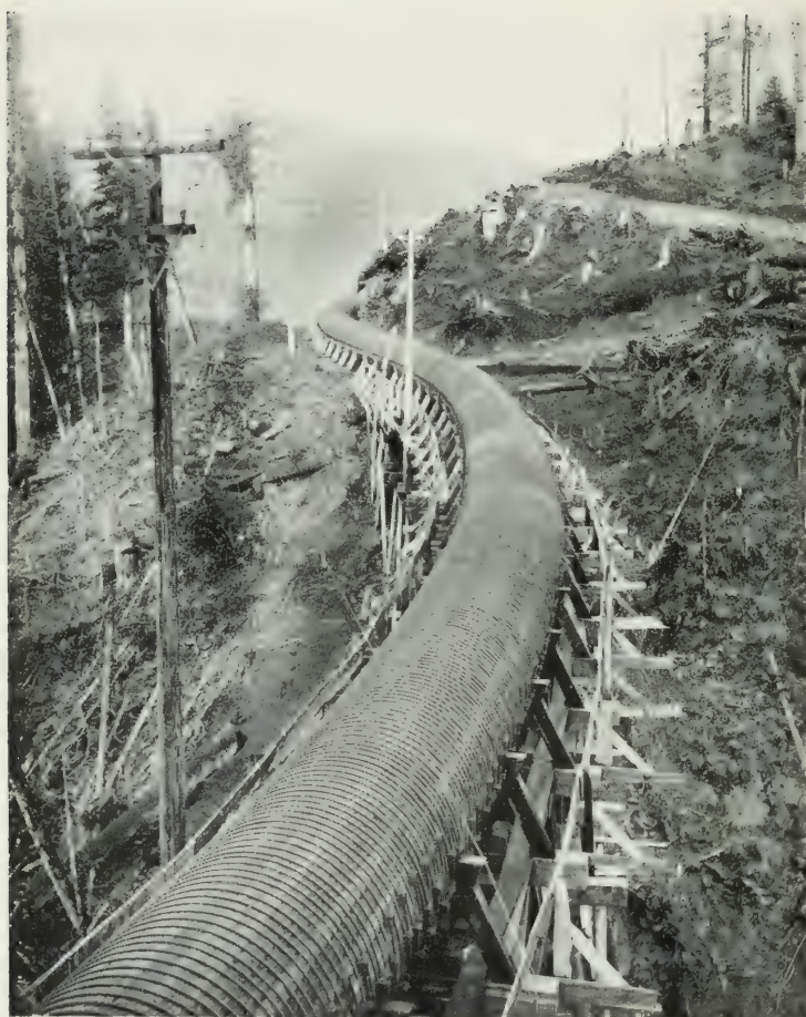
FIG. 23. 4-MILE PIPE LINE OF WOODEN STAVES : FOR POWER.
